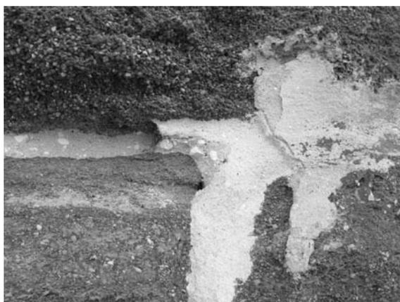
**Fig. 1.** Detail of a mortar joint in an eighteenth-century masonry wall, showing three layers of mortar. Multiple layers of mortars of different compositions and ages complicate the process of taking samples for mortar analysis. Images by the author, unless otherwise noted.
