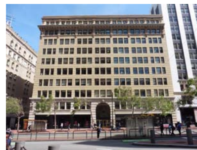
Monadnock Building. Photo by Jason Wright.
