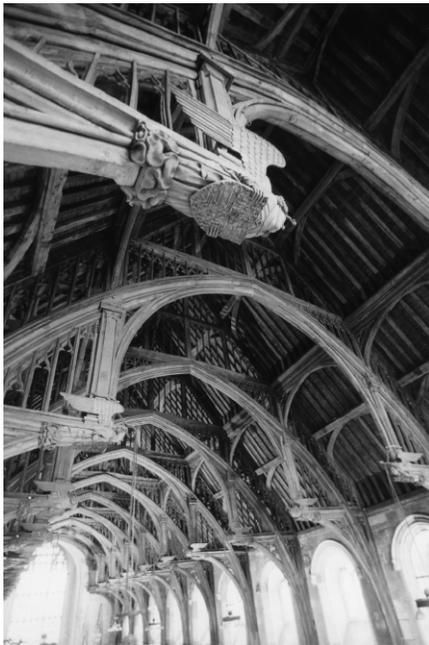
Fig. 1. Westminster Hall roof, the Palace of Westminster, British Parliament, London, complex historic structure and materials. The hammer-beam oak roof of 1399 AD by Richard II's master carpenter, Hugh Herland, spans 68 feet (20.7m), is 240 feet (73.2m) long, and weighs 836 tons, including the wooden construction and lead-sheet covering. © UK Parliament [www.parliament.uk](http://www.parliament.uk).
