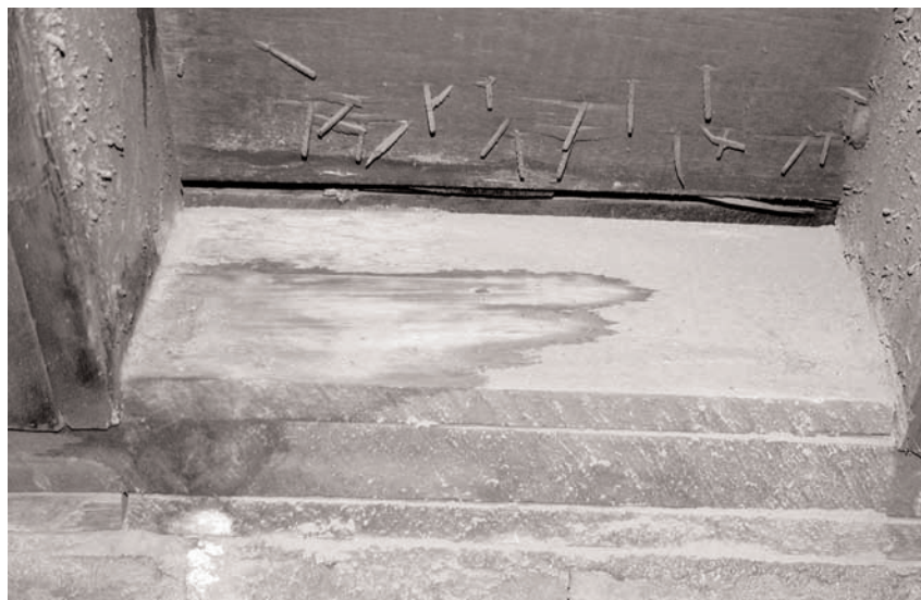
Fig. 1. Moisture stain on a sill plate on top of a masonry dome. All photographs by the author.
