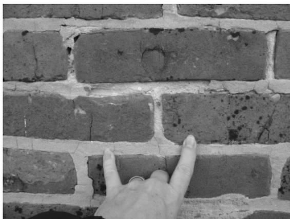
**Fig. 1.** Image of an historic brick masonry wall that has had a new mortar smeared over the existing original instead of being raked out and repointed properly. Preliminary field assessment by an experienced preservation professional is essential for defining a mortar-analysis program. An inexperienced preservation professional might mistake this construction as having different pointing and setting mortars. All illustrations by the author.
