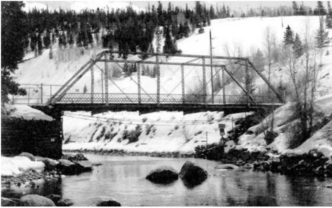
Fig. 2. Blue River Bridge over the Blue River, near Silverthorne and Dillon, Colorado. This steel Pratt truss has five bays and an 80-foot (24-meter) span. It is believed to have been built in about 1895 as Two-Mile Bridge near Breckenridge, Colorado, and moved to this site at a later, but unknown, date.
