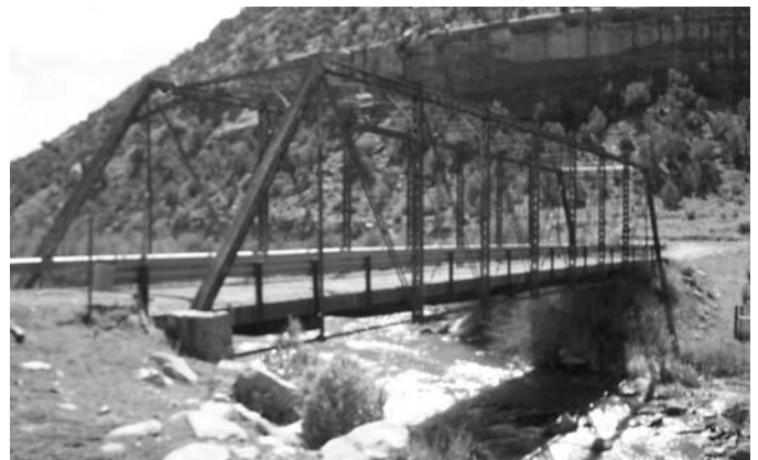
Fig. 5. San Miguel Bridge over San Miguel River in western Montrose County, Colorado. This wrought-iron bridge with a 142-foot (43-meter) span was built in 1886. In 1964 its timber deck and stringers were replaced with steel stringers with semicircular segments of corrugated-metal pipe that bear on the bottom flanges of the stringers, topped with gravel roadbed.
