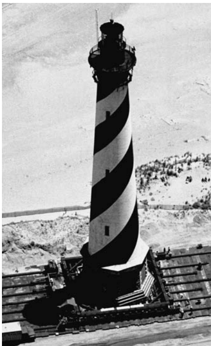
Fig. 1. Cape Hatteras lighthouse being moved. Courtesy of Western Carolina University.
