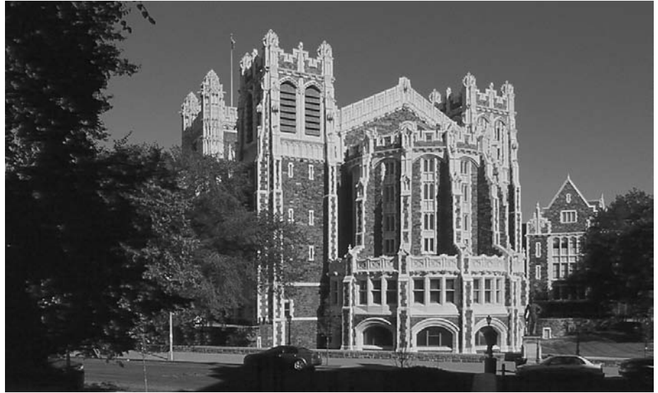
Fig. 4. Shepard Hall, City College of New York. Courtesy of Robert Silman Associates.
