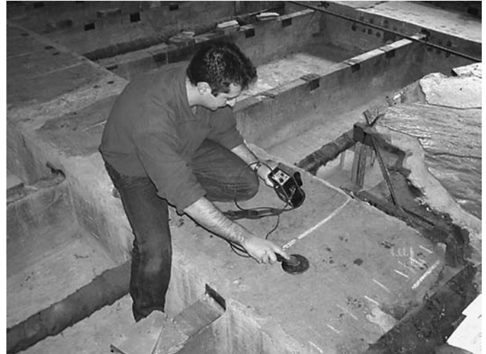
Fig. 9. Fallingwater, using radar as a nondestructive evaluation technique to find reinforcing bars in concrete beams. Courtesy of Robert Silman Associates.
