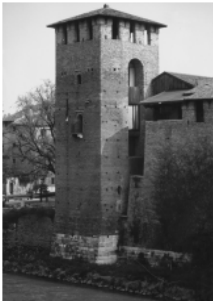
Fig. 1. At the Castelvecchio in Verona, Italy, architect Carlo Scarpa negated the defensive nature of the castle by removing a vertical section of stone from the protective wall and cutting it loose from its corner tower to emphasize its height and construction. Photograph by Platt Byard Dovell White, Architects.
