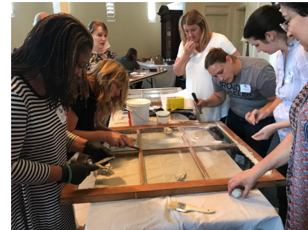
Students reglazing window sash at the 2017 Preservation Training for Museums and Cultural Institutions event hosted by the Florida Association of Museums Foundation. Photograph courtesy of the Florida Association of Museums Foundation.
