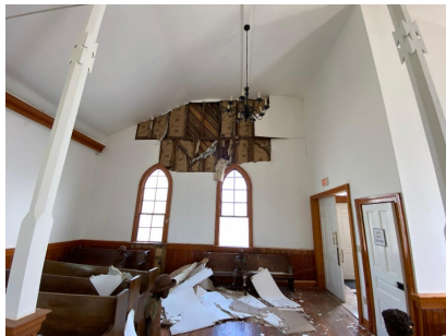
Damage to gable end wall of the Antioch Baptist Church, Whitney Plantation. Courtesy of APT DRI.
