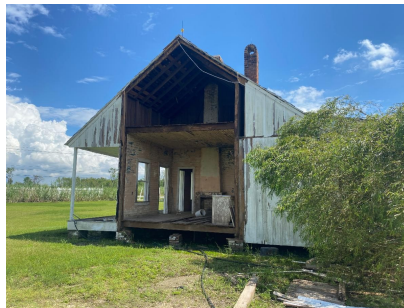
Damage to gable end wall of the Milaret Manager House, Whitney Plantation. Courtesy of APT DRI.
