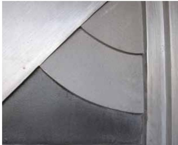
Fig. 1. Satin finish is in the upper left corner and right side. Sandblasted finish is on the upper right and middle. A replicated deplated finish is on the bottom. Samples are from a subway station in New York, New York. Images by the authors unless otherwise noted.
