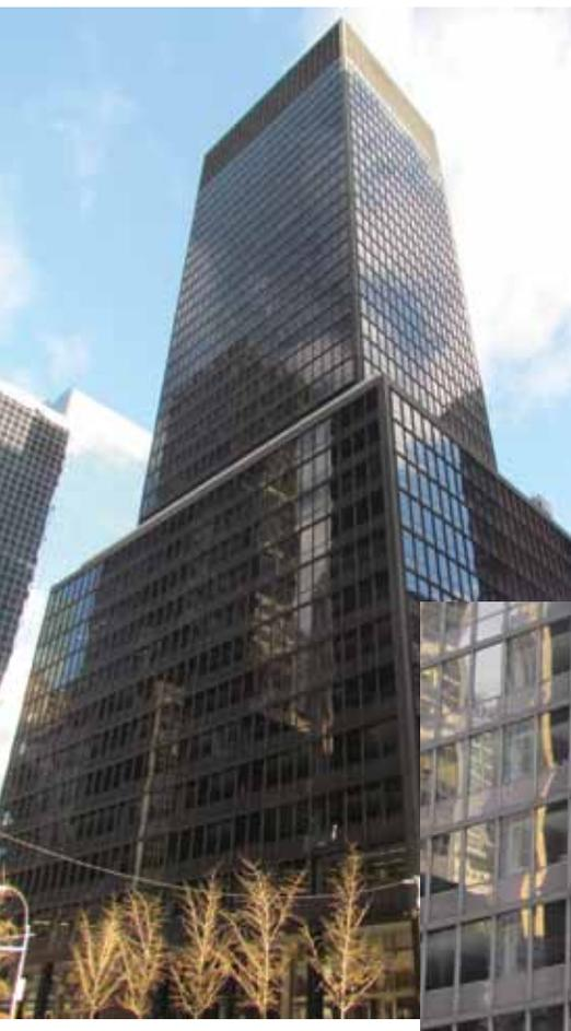
Fig. 8. U.S. Plywood Building, 777 Third Avenue, New York City, designed by William Lescaze and built between 1961 and 1963. The facade is clad in glass and dark anodized aluminum.
