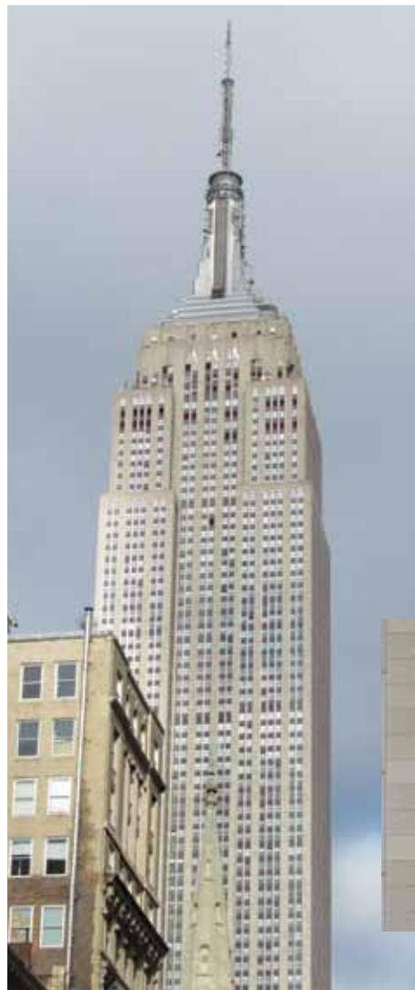
Fig. 6. Empire State Building, New York City, designed by William F. Lamb and built between 1929 and 1931. Aluminum spandrel panels were designed with a deplated finish.
