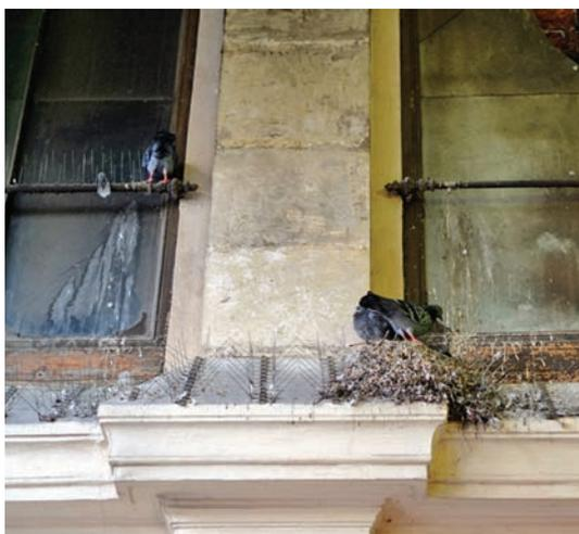
Fig. 2. Passage Vendome, Paris 3e, France, showing soiling of buildings caused by nesting pigeons. Note the inefficacy of the spikes.
