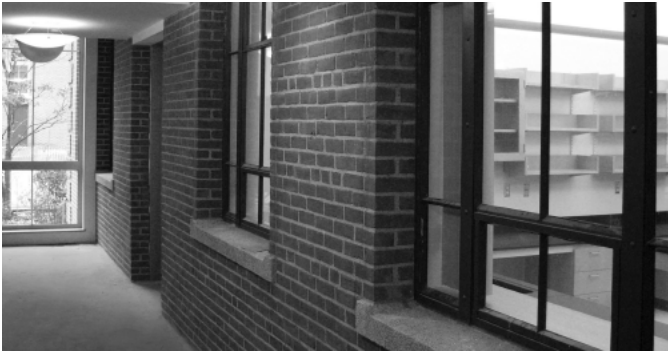
Fig. 5. James Hall, University of New Hampshire, 2009. The steel windows from the original exterior envelope were refinished within the newly enclosed circulation area in the addition, offering views from the corridor to the laboratories in the existing building.
