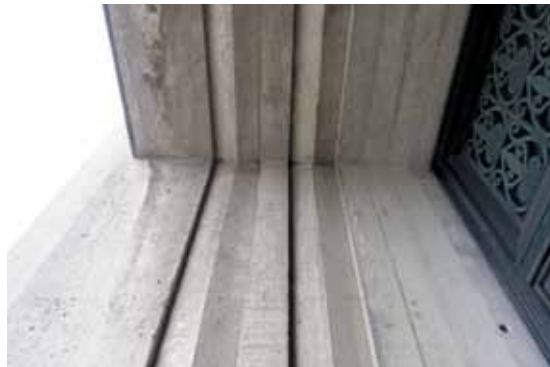
Fig. 4. Smooth-form concrete finish.
