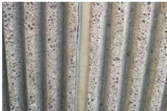
Fig. 6. Board-formed concrete finish.
