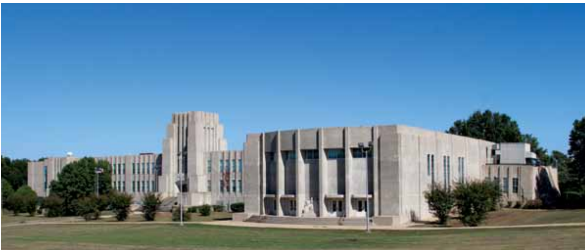
Fig. 1. Exposed architectural-concrete facade and concrete elements at the Bailey School in Jackson, Mississippi, designed by architect A. Hays Town and built in the 1920s. Photograph 2016. All photographs by the authors unless otherwise noted.
