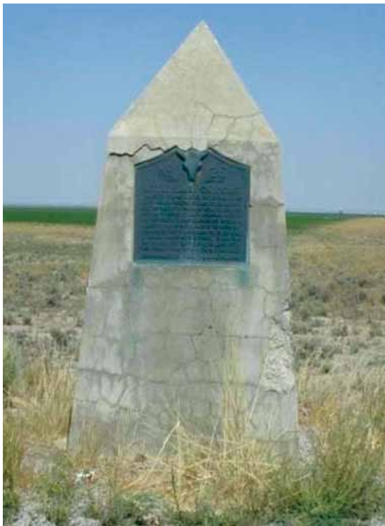
Fig. 9. Freezing- and thawing- related distress at a historic exposed-concrete monument, Wyoming, 2008.
