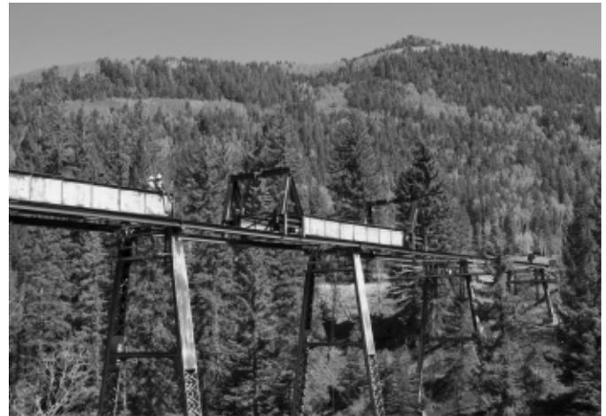
Fig. 7. A temporary gantry was used by the contractor for removing girder segments and installing new girder segments. The gantry rolls on a temporary beam that also served to provide longitudinal bracing for the structure during construction. Photograph by Roger Hogan for CTSRR.
