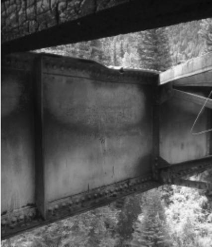
Fig. 3. Fire damage at a girder. Distortion at the upper portions of the girder flange can be seen. Paint has been burned off the upper flange and has been discolored at the upper part of the web. Photograph by Roger Hogan for CTSRR.
