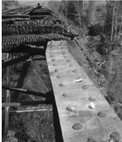
Fig. 4. Fire damage. The riveted plate girder is distorted, ties are burned, and track displaced. Photograph by Roger Hogan for CTSRR.
