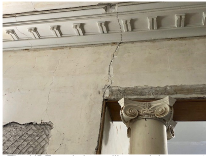
The NDE workshop will spend day one at the Willowbank School in Queenston, Ontario, where participants will experiment with NDE equipment on the historic fabric of the 1830s Greek Revival mansion.
