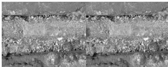
Fig. 10. Stereo images of an eroded mortar joint.
